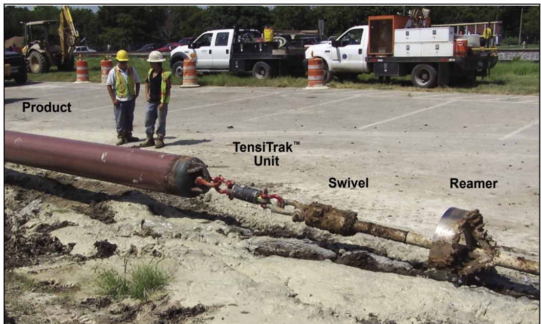
TensiTrak™ assembly with 18-in. (457-mm) steel casing ready for installation in Texas.
