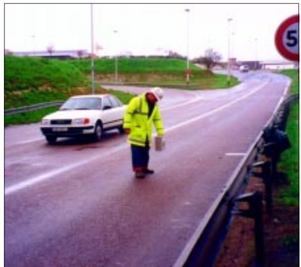
Tracking the drill head under a French motorway.
