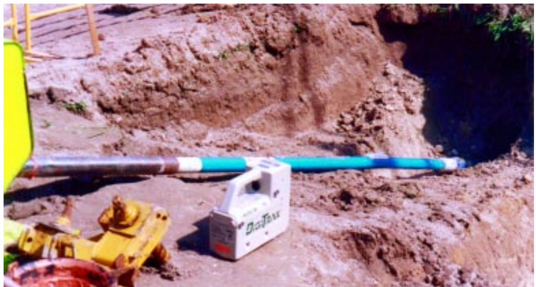
The drill string heading into the ground at the starting pit.
