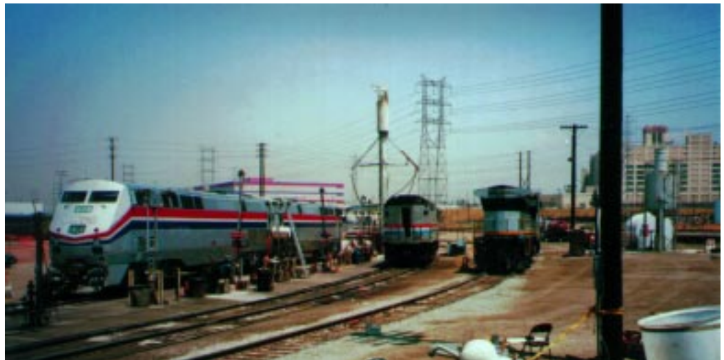
The Los Angeles Amtrak roundhouse switching station proved to be a very difficult site for underground locating.
