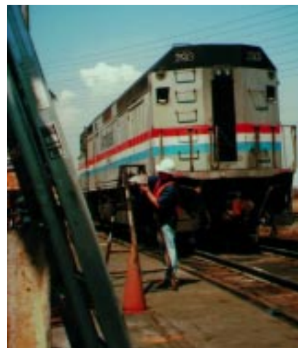
Placing DigiTrak receiver on ladder to minimize below-ground interference.
