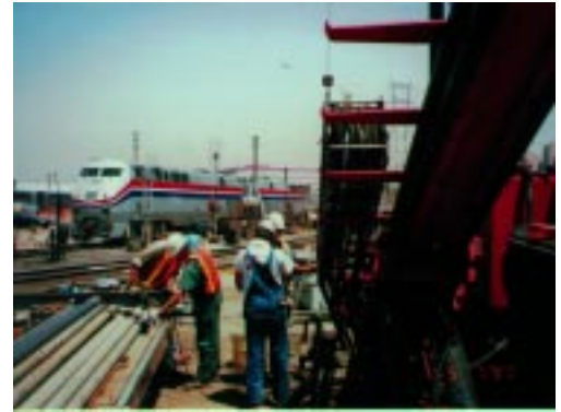
Setting up the bore at the start of the run.
