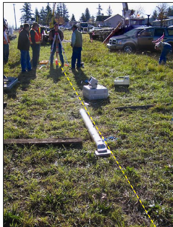
Aligning Drill to Marked Bore Path
