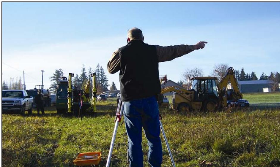
Aligning Drill to Marked Bore Path
