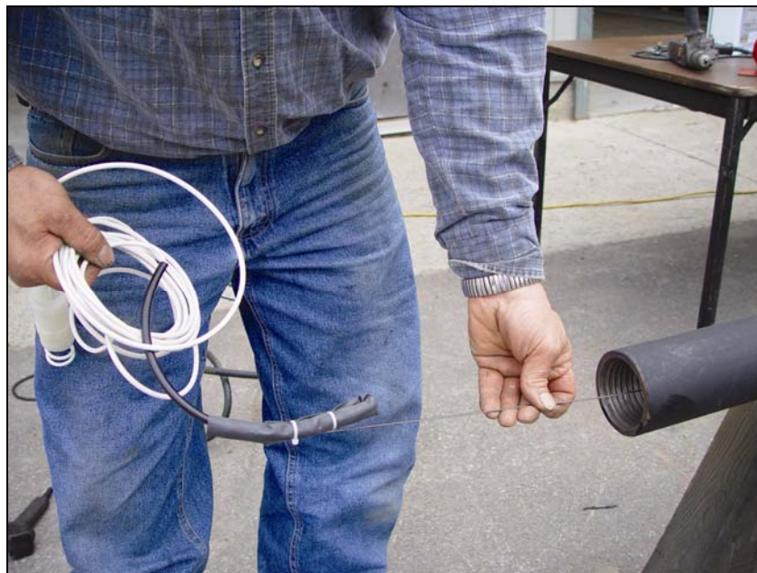
Attaching Box End to Fish Tape to Pull Through Rod
