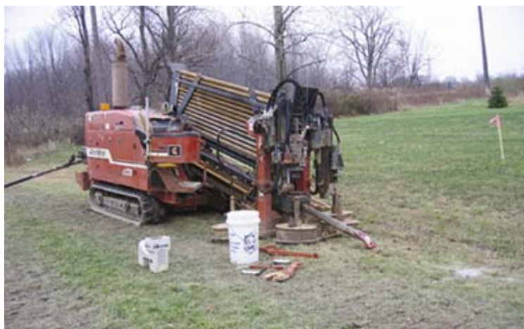
Figure 8. The drill ready to launch the pilot bore
