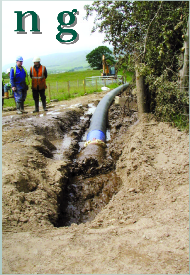
The pullback of the 16-in. (400-mm) product pipe commences.
